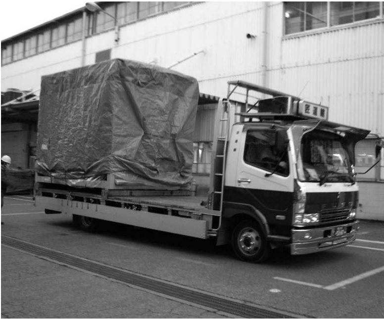
Figure 4. A completed, wrapped room module on the truck, ready to haul to the building site. Modules are designed not to be oversized loads on most Japanese streets and highways; special escorts are unnecessary.
